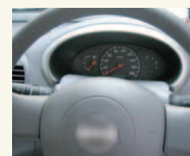
Fixing sound absorption materials around instrument panels
