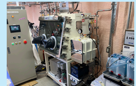
Formic acid production equipment
